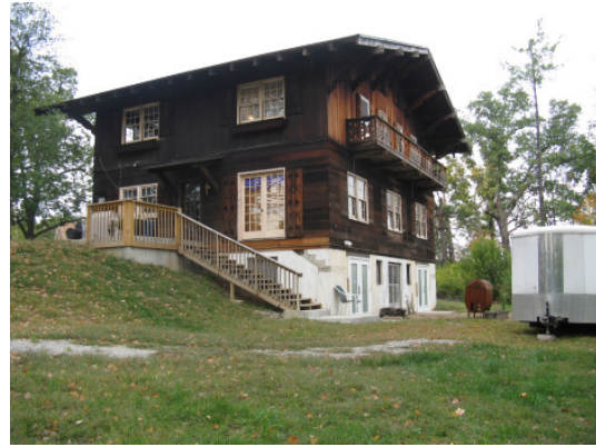
View looking northwest into the site
