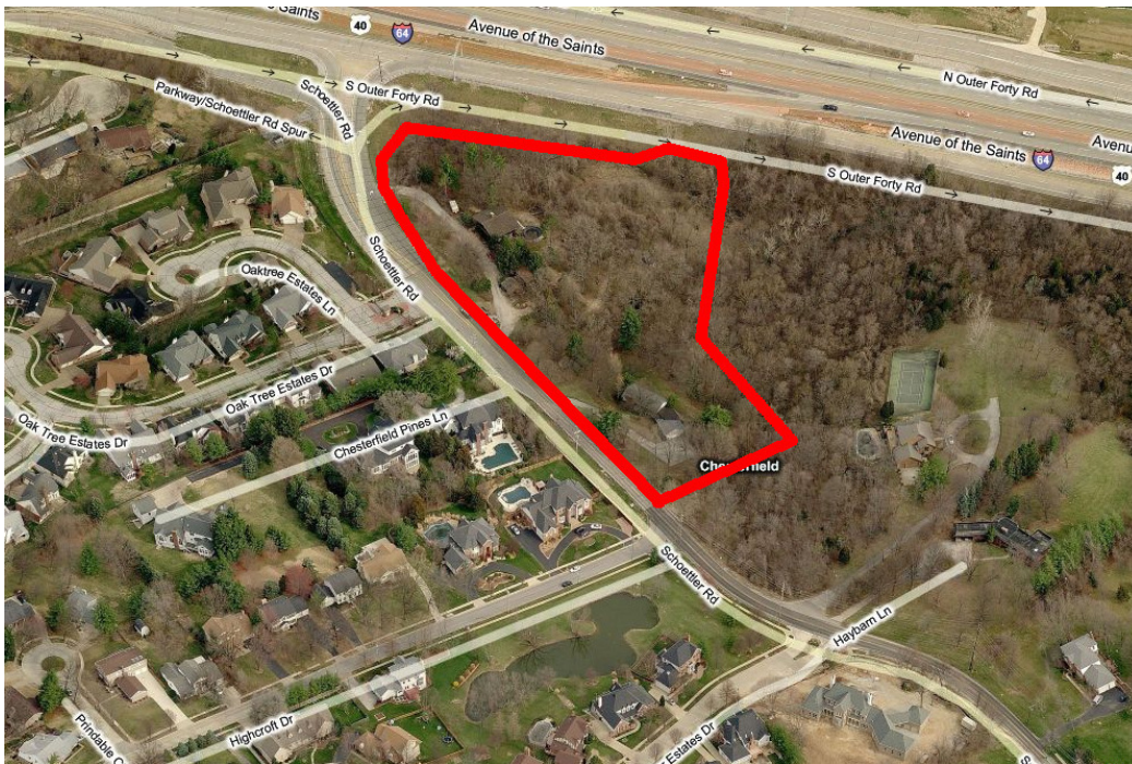
Aerial View of the site
