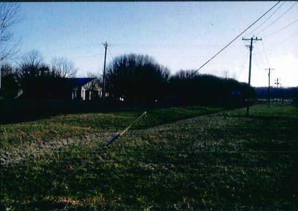
VIEW LOOKING EAST
