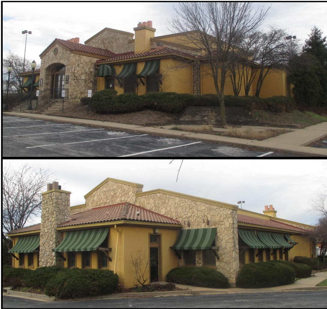
Figure 3. Existing Structure Photos
