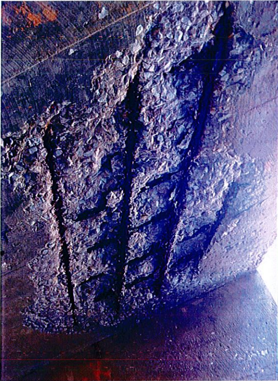
PHOTOS C,D: ADVANCED DETERIORATION OF TOP SLAB OF CULVERT
