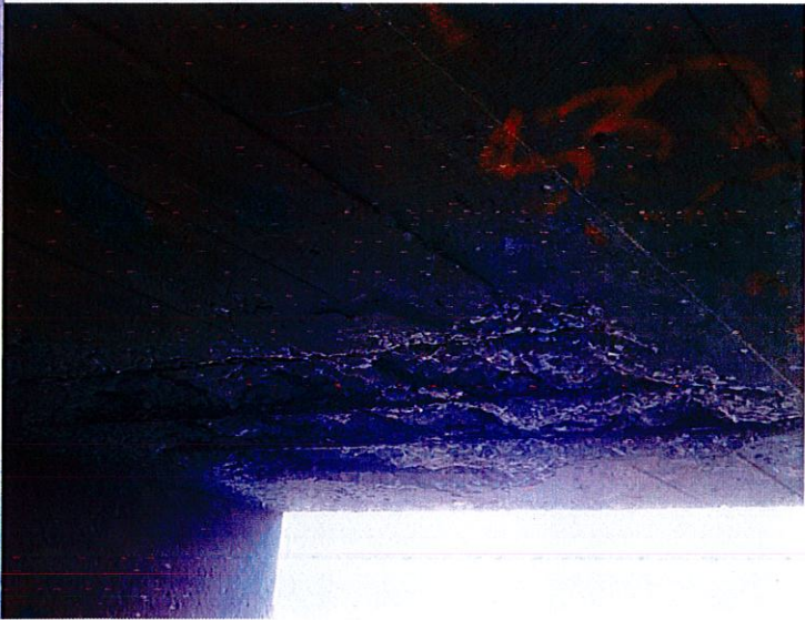
PHOTOS C,D: ADVANCED DETERIORATION OF TOP SLAB OF CULVERT
