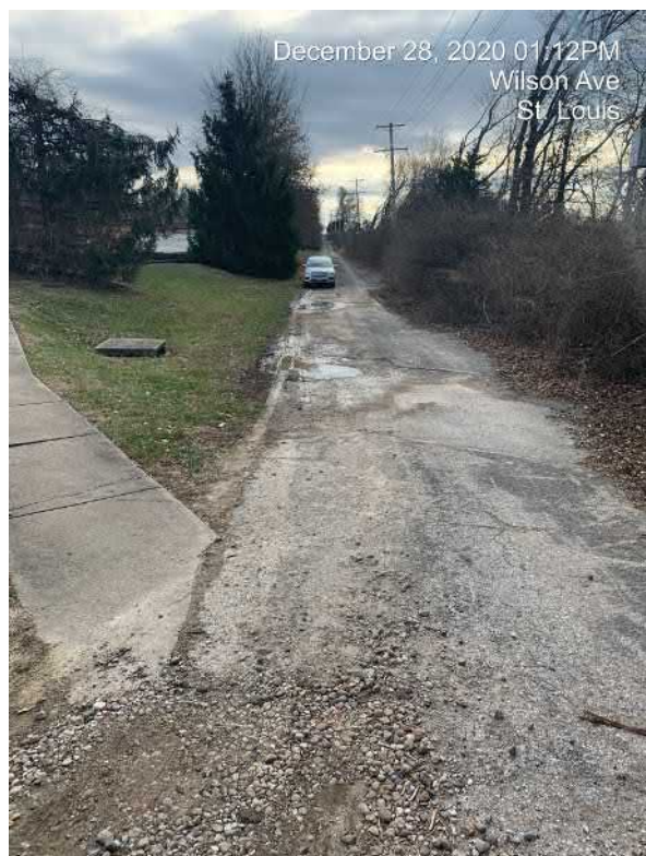
Existing Access Drive to 2153 Wilson Ave.
