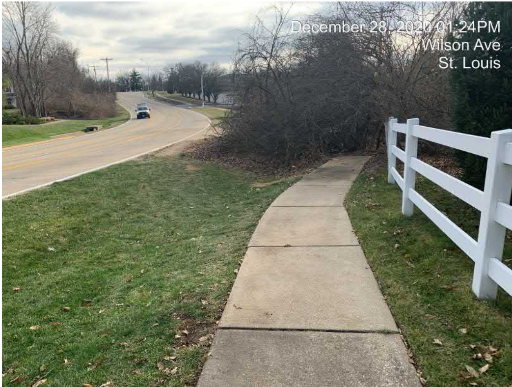
Existing Sidewalk Termination Point along Sea Beauty Farm.
