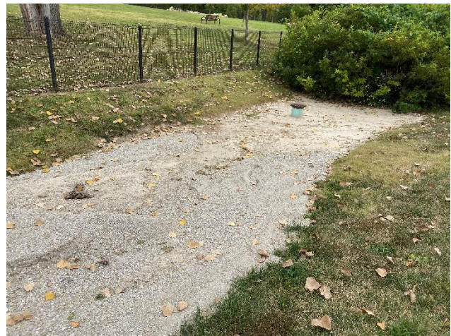
Figure 9 – Bioretention basin on the inside of the loop, between the fenced dog park and North Trail, from the western leg, facing southwest.
