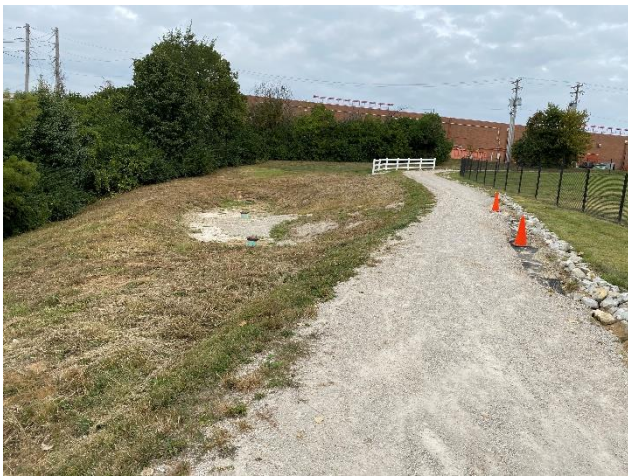
Figure 8 – Bioretention basin as northwest corner of the North Trail, from western leg, facing north.
