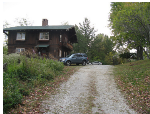
View looking south into the site
