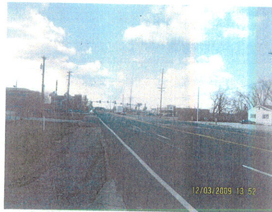
View Looking west along Chesterfield Airport Road.
