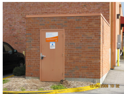
Existing equipment room
