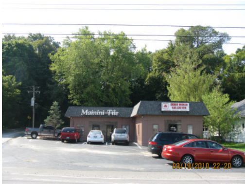
View looking South into the site from Old Chesterfield Road
