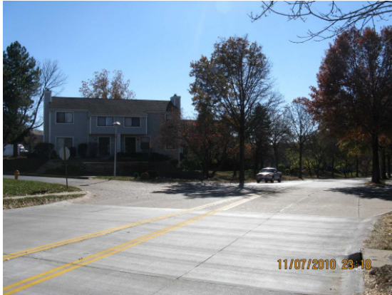
View looking at an apartment building.
