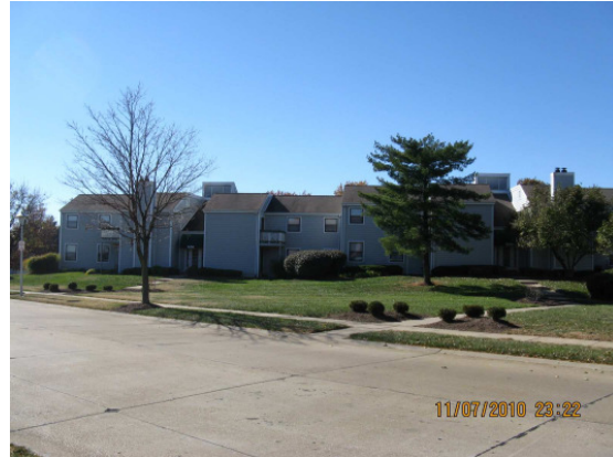
View Looking at an apartment building.
