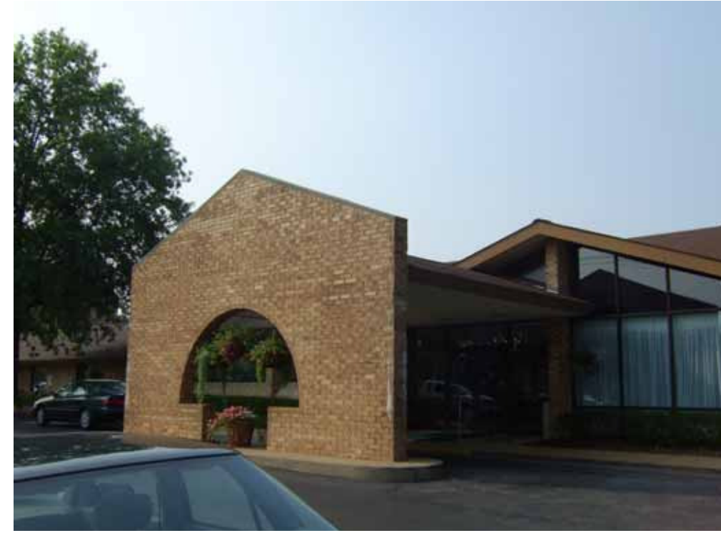
DELMAR GARDENS OF CHESTERFIELD (EXISTING EAST OF FACILITY)
