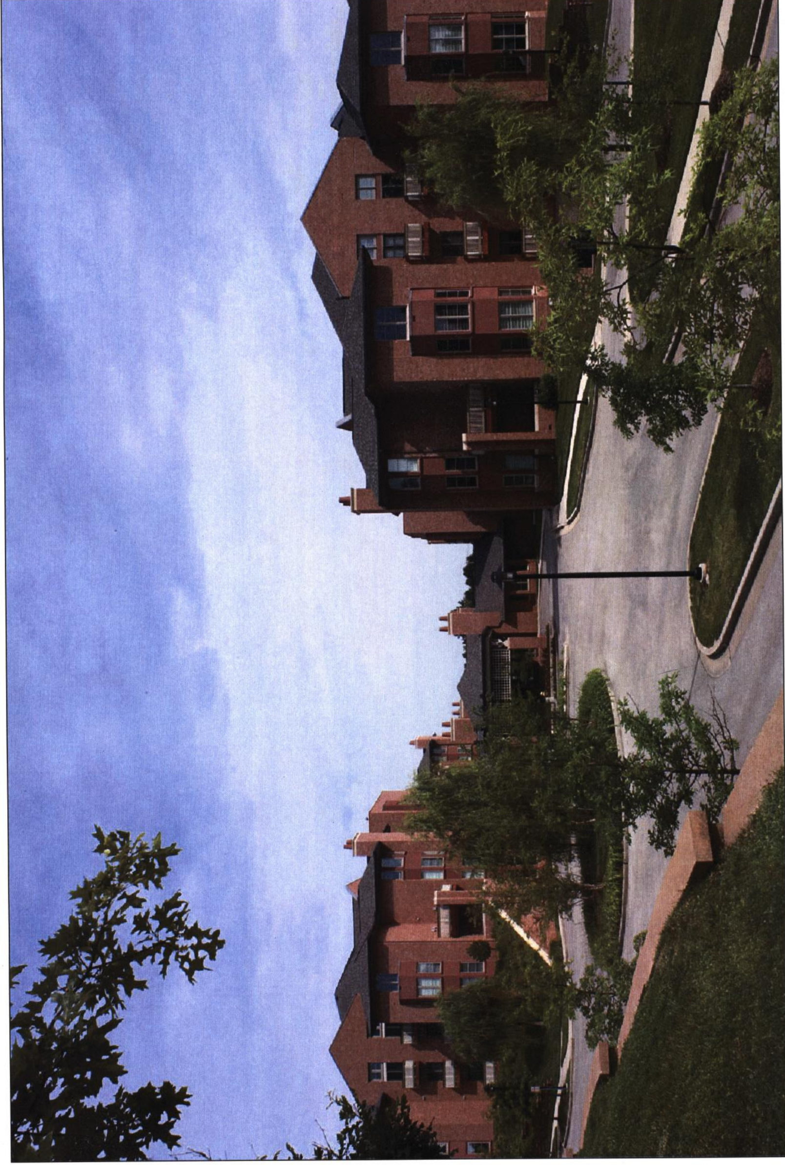
Phase I & II - South Entry (Buildings A & E Elevations Similar)
