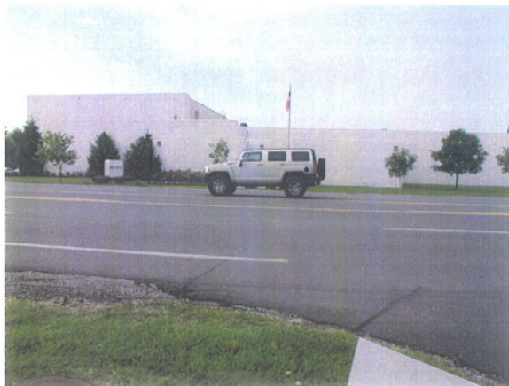
Looking south, across Chesterfield Airport Road.
