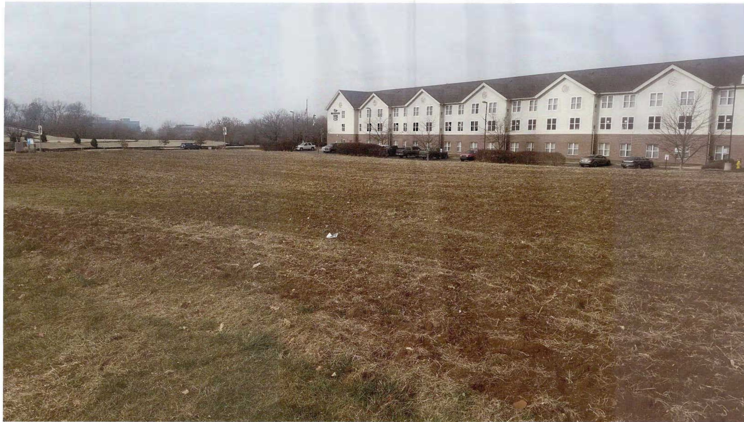
View from site looking Northwest
