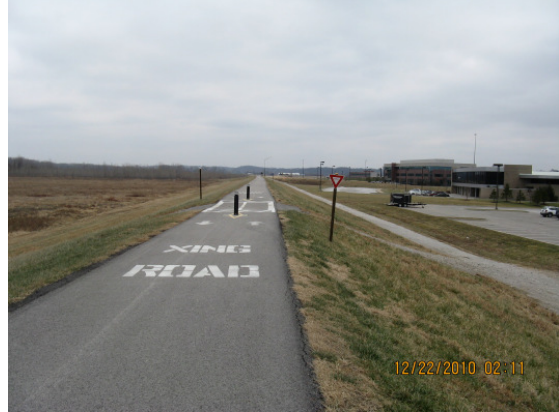
View looking east along the top of the levee trail
