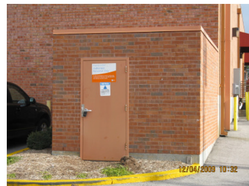
Existing equipment room
