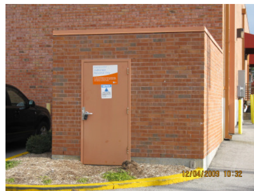
Existing equipment room
