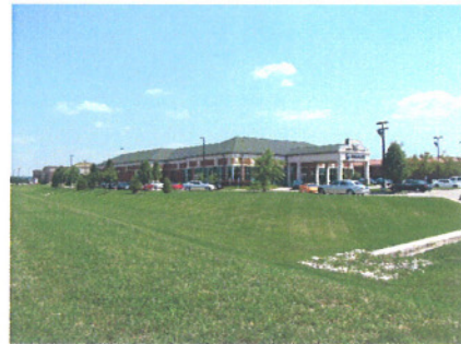
VIEW FROM LOCATION "C" LOOKING SOUTHEAST
