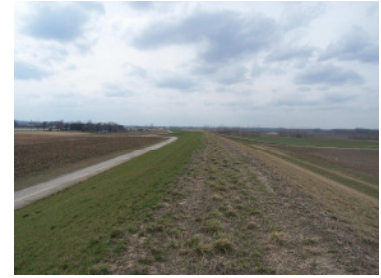
LOCATION "B" VIEW LOOKING WEST
