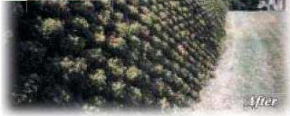
Apartment community tie wall replacement
