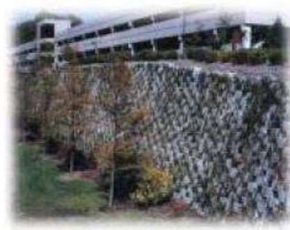
Corporate headquarters, gravity wall up to 18 feet tall.
